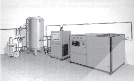
Fig. 8.8 : Compressor station with screw compressor, compressed air receiver, refrigeration compressed air dryer and filter system
